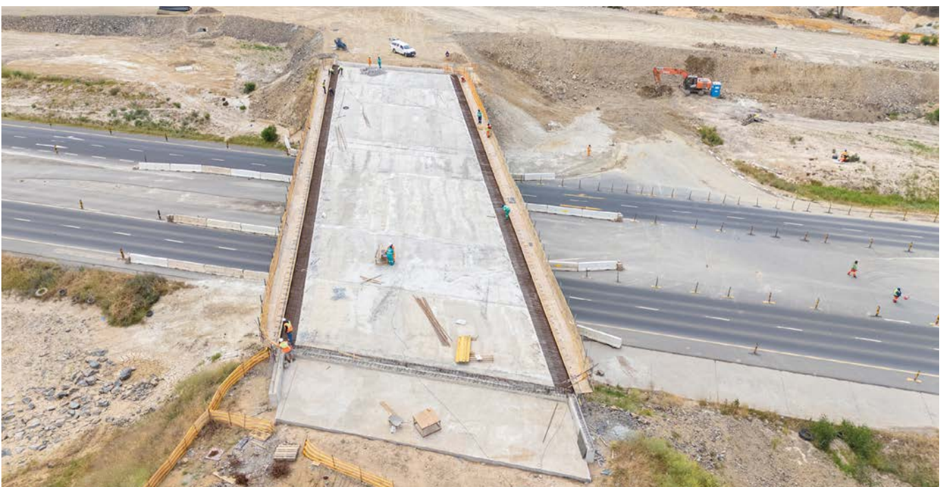
The in-situ slab was constructed in stages, ensuring that the deck is continuous over diaphragms, with a sidewalk and balustrade.
