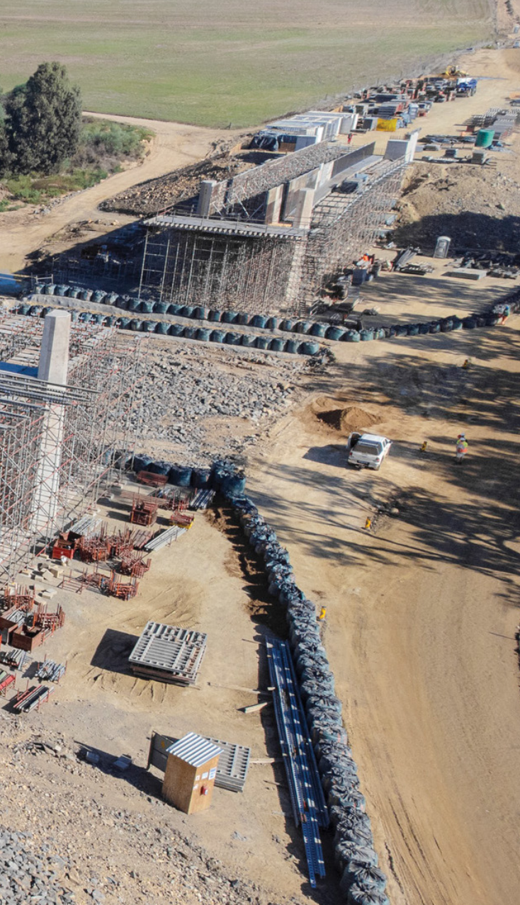
A temporary stressing design allowed for framework to be removed from the first two outer decks and to construct the central deck before stressing the whole deck as one.
