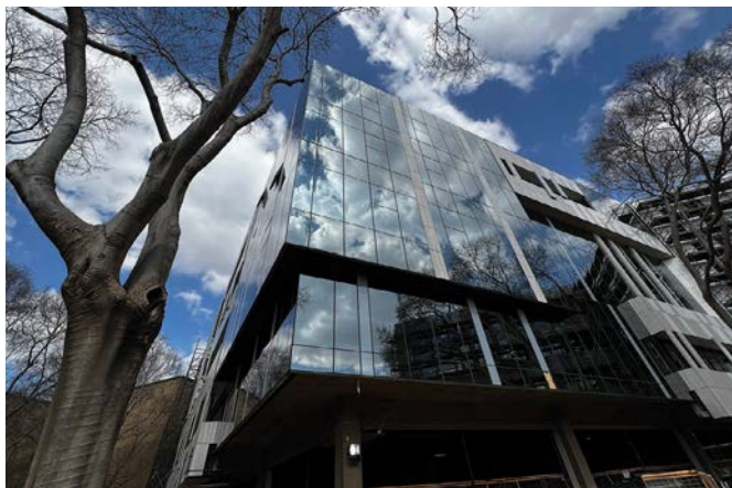
A standout feature of the refurbished Compensation Fund House will be its striking new façade which incorporates a modern curtain walling system for a sleek contemporary look.
