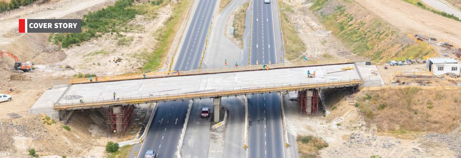
The B6113 is a four span bridge designed with three piers consisting of trestle beams supported on 750 mm diameter friction-type piles.
