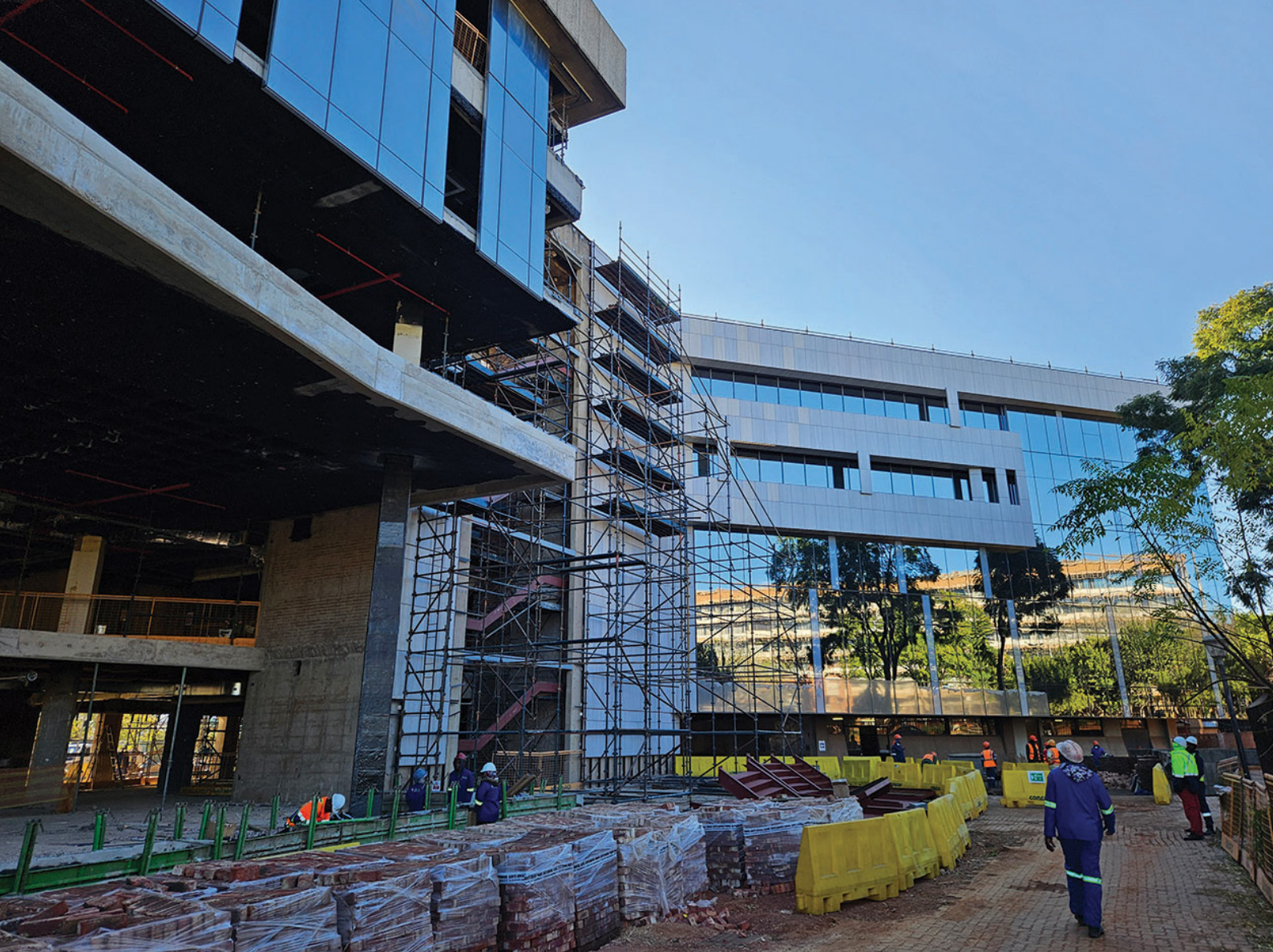
Façade works at an advanced stage with the installation of unitised panels nearing completion.
