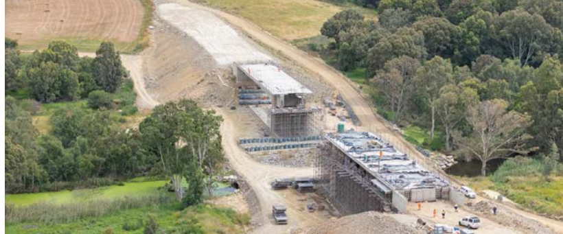
A temporary stressing design allowed for framework to be removed from the first two outer decks and to construct the central deck before stressing the whole deck as one.
