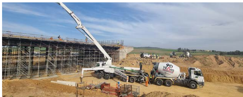
AfriSam used 25 to 30% fly-ash mix to help control the heat of hydration and to contribute to durability.
