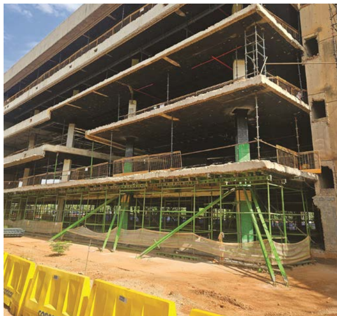
Structural remedial works and partial demolition underway at Compensation Fund House as part of the building's refurbishment programme.
