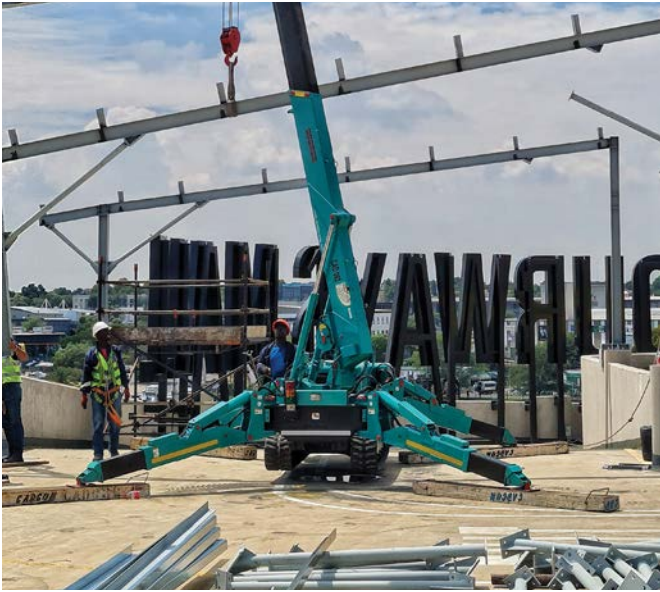
Left: Lightweight construction methods are being employed with the use of spider cranes and dumpers that are suitable for the project's weight restrictions. Right: The rehabilitation of the 8 000 m 2 access ring road is key to the successful functioning of the mall by ensuring access of visitors to the mall.
