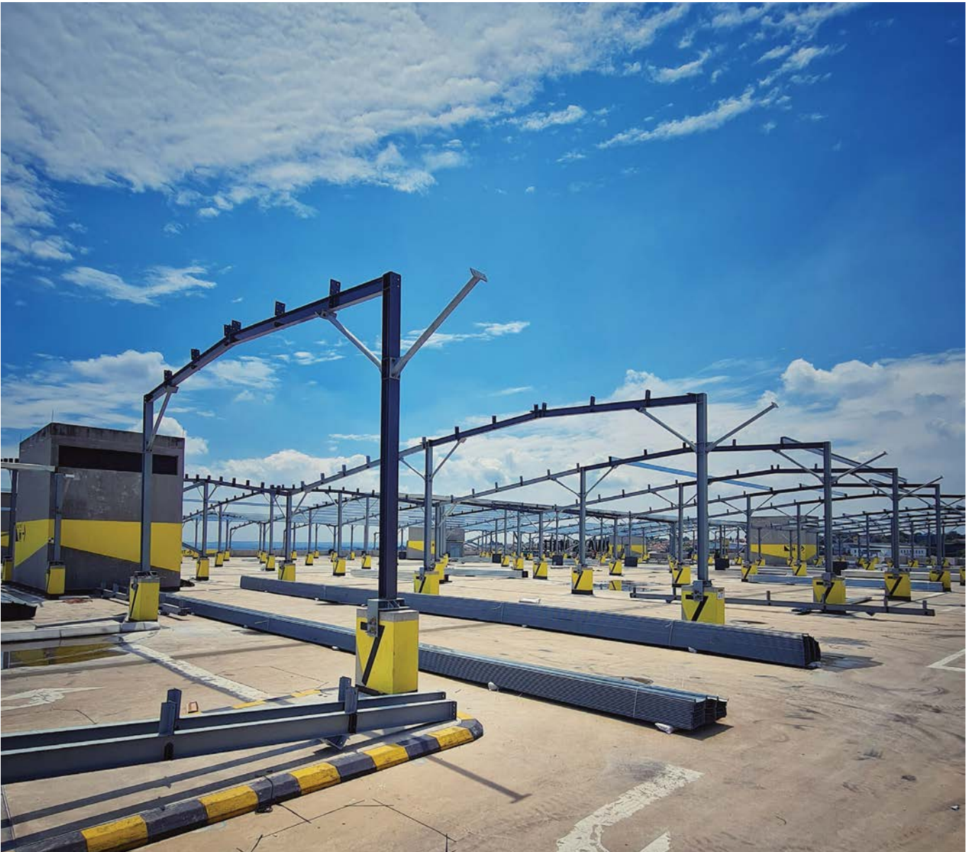
Concor is providing the steel structure to support the installation of a PV installation that will assist with the mall's sustainability and energy aspirations.
