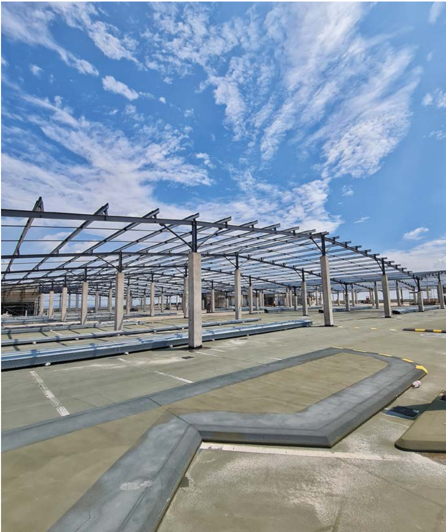
This fast track upgrade project started in October and forms part of the Fourways Mall Repositioning initiative and involves covering 50 000 m 2 of the roof parking on level 7 with a roof.
