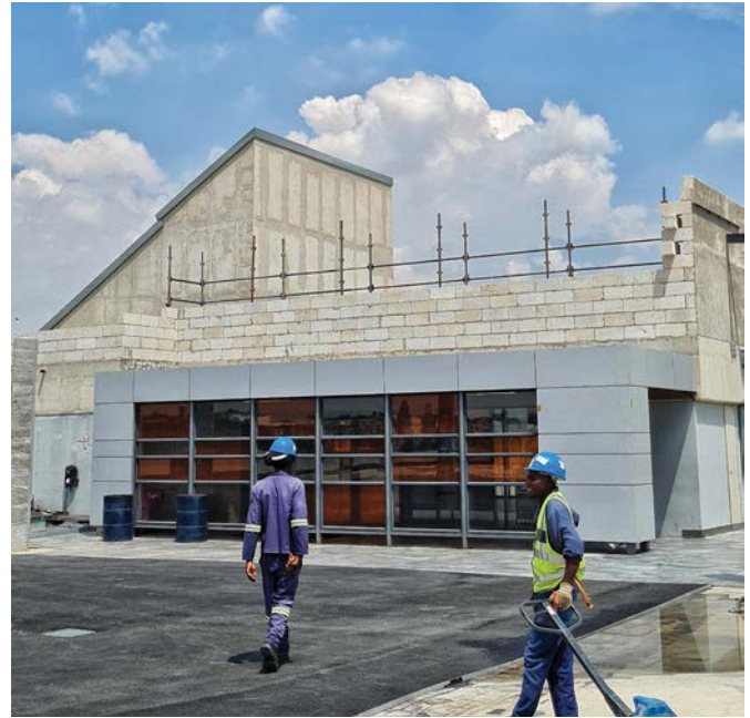
Left: The initial plan was for the roof to have a physical curved structure which would have increased cost and weight, but the roof structure makes use of straight trusses and it is adjusted to allow a sloped finish. Right: Lightweight Hebel bricks are being used to build walls around the lift lobbies and will be used for signage to ensure that visitors can orientate themselves when parking on the roof.
