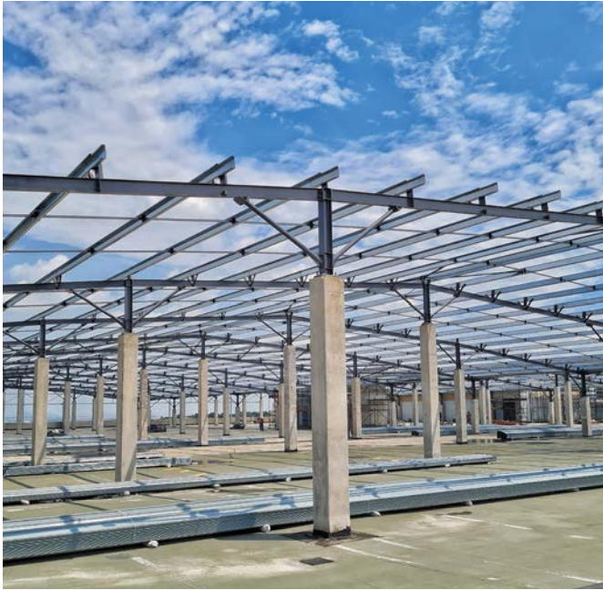
Left: The initial plan was for the roof to have a physical curved structure which would have increased cost and weight, but the roof structure makes use of straight trusses and it is adjusted to allow a sloped finish. Right: Lightweight Hebel bricks are being used to build walls around the lift lobbies and will be used for signage to ensure that visitors can orientate themselves when parking on the roof.
