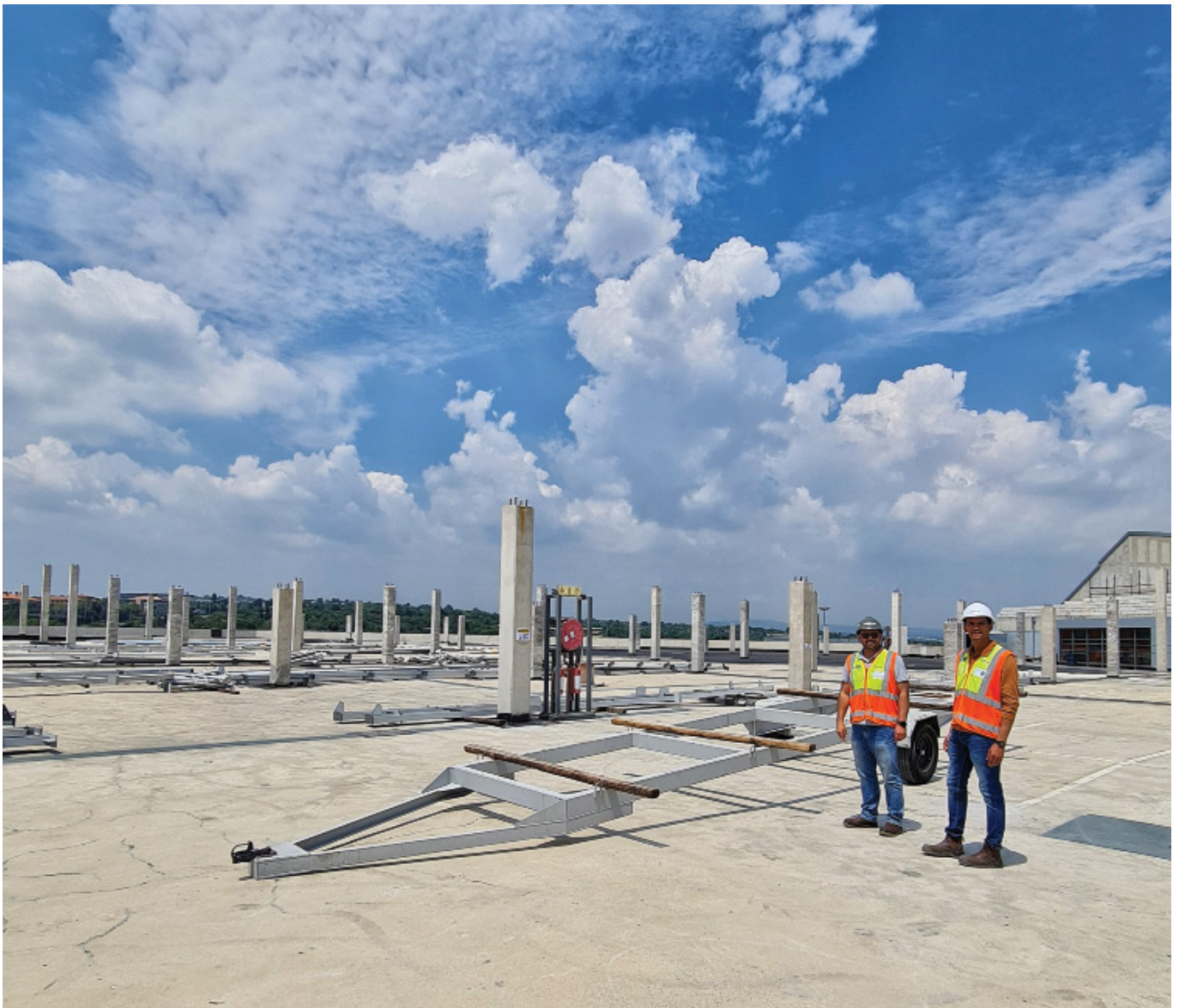
The trailer uses to transport structural steel from street level was specifically built for the project.
