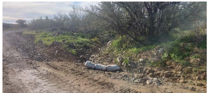
A sandbag silt trap is installed at the watercourse crossing on the Karreebosch Wind Farm facility to safeguard the environment during construction.
