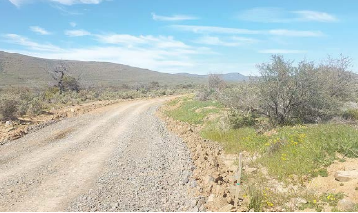
Topsoil is preserved along a road servitude at the Karreebosch Wind Farm facility, ensuring environmental care during construction.
