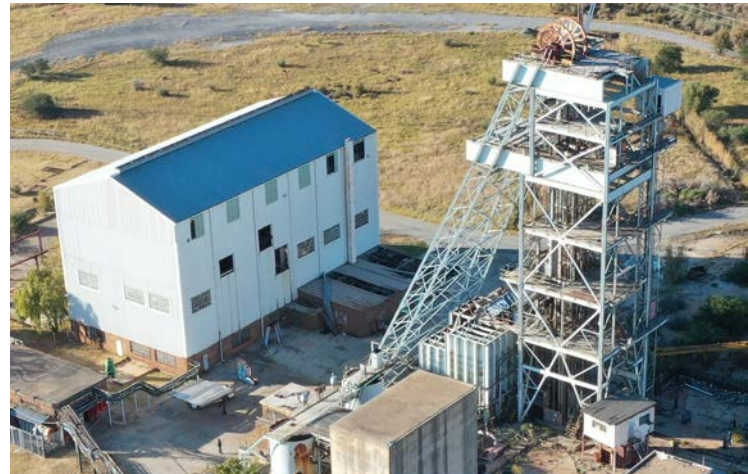
Rehabilitation & demolition of Beatrix 2 shaft & outbuildings for Sibanye Stillwater.
