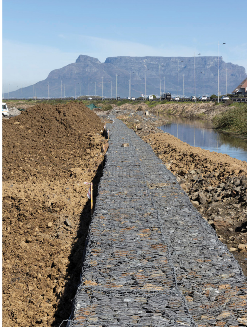
About 15 000 tonnes of large stones of up to 200 mm in size are being delivered for the gabion baskets.
