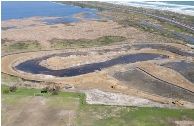
A 460 metre long secondary treatment canal will ensure that finer matter also drops out of suspension as the water passes through.
