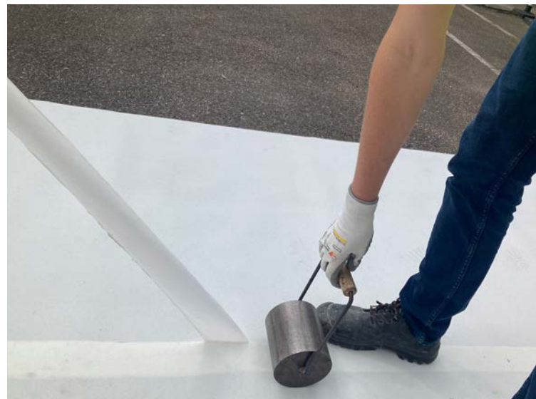
PREPRUFE® 120S provides fully bonded waterproofing that effectively prevents water migration.
