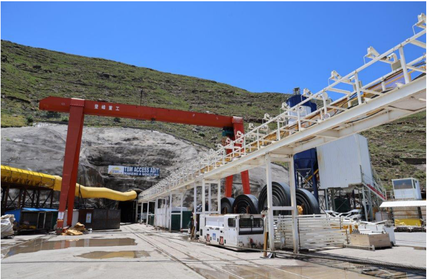
Polihali Dam incorporates a 5 m-diameter TBM tunnel with intake works, gate shaft, and outlet connecting to Katse Reservoir.
