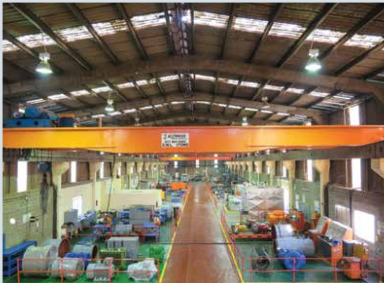
Marthinusen & Coutts' facility in Kitwe, Zambia.
