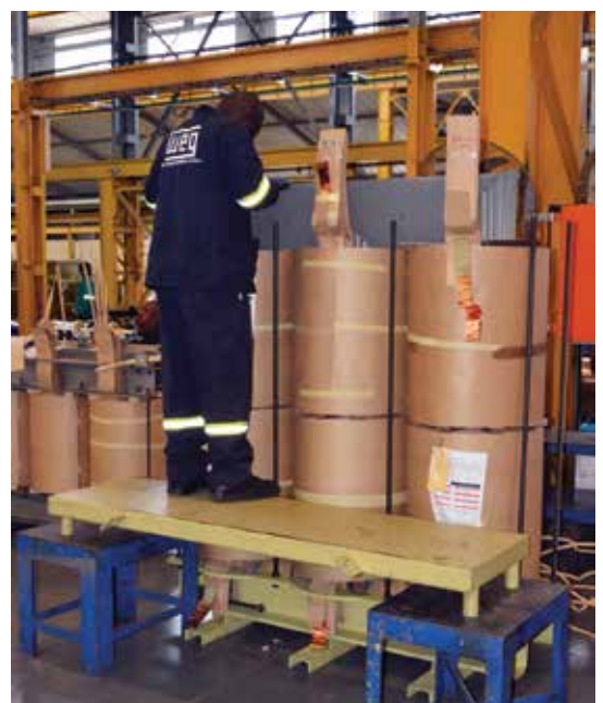
Active part assembly on a WEG PV transformer.
