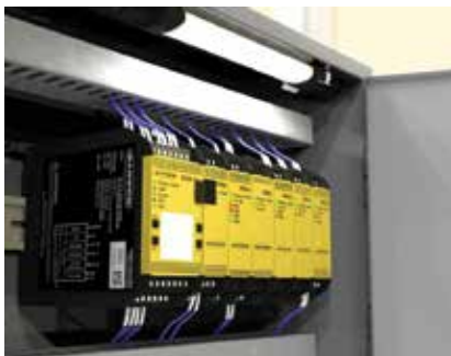
Turck Banner's SC-XM3 external drive allows for easy setup and consistent configuration of safety controllers.
