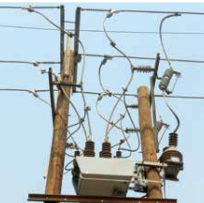
Dual pole overhead line assembly.
