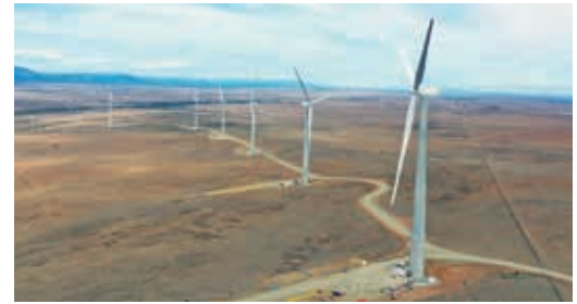
Now operational, Nxuba wind farm in the Eastern Cape is expected to generate 460 GWh of energy annually.
