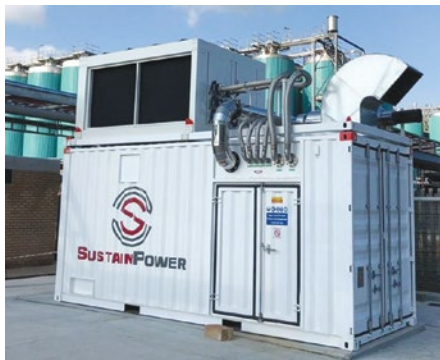
Containerised CHP unit at Distell Springs.
