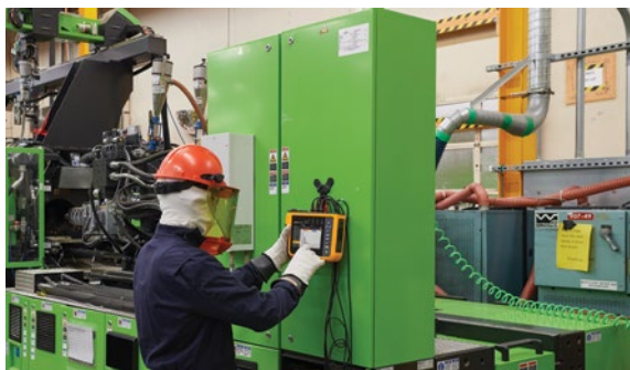
The Fluke 1770 Series power quality analysers capture more than 500 power quality parameters by default, tracking critical power quality events.
