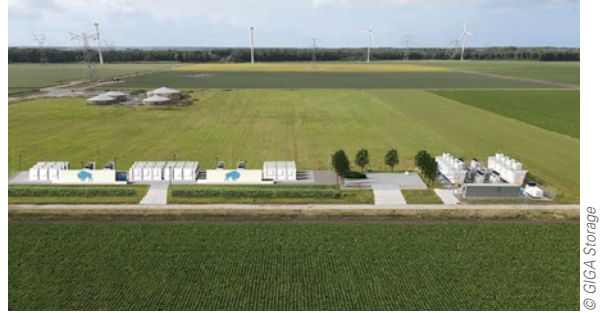
The 25 MW/48 MWh Buffalo battery in the Netherlands will support grid stability.
