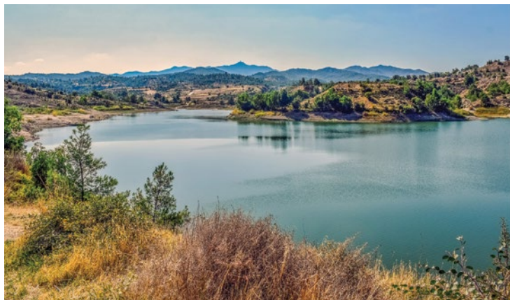
Monitoring remote reservoirs and controlling water pump stations can become costly using wireless telemetry relying on licensed band radio frequencies.
