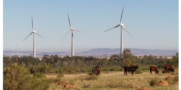
Gouda wind farm in the Drakenstein municipality, Western Cape, has 46 wind turbines mounted on 100 m high concrete towers, locally manufactured.
