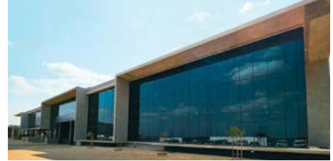
The first phase of Teraco's JB4 campus includes 8 000 m 2 of data hall space, with 19 MW of critical power load.
