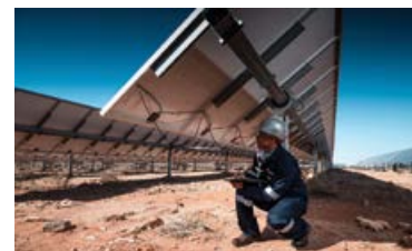
The Kenhardt project will have a total solar capacity of 540 MW and battery storage capacity of 225 MW/1 140 MWh.
