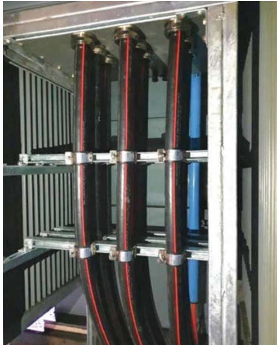
Cleat installation: securing, fixing and routing electrical cables.
