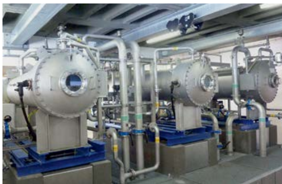
In pressurised reactors, electrical energy is applied to convert oxygen into ozone which is used in the production of safe drinking water.
