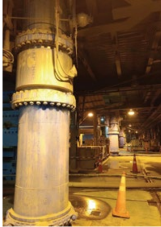
KROHNE flowmeters are used for measurement of slurry feeds to hydrocyclones.
