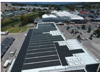
The micro-grid system combines solar PV panels, battery energy storage and storage converters.
