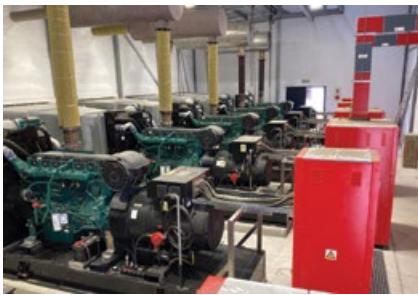
The 550 kVA gensets in the client's generator plant room on site.
