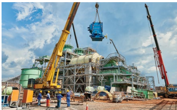
One of the WEG high voltage motors being lifted into position on site at Kamoa-Kakula.
