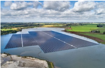
The Bomhofsplas photovoltaic system, which floats on a gravel quarry near Zwolle in the Netherlands.
