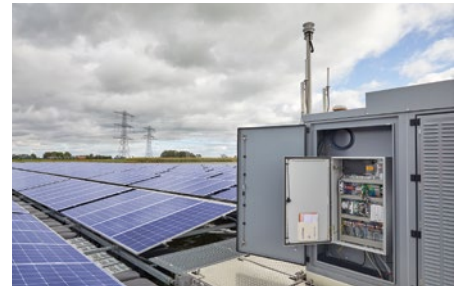
Omnidirectional antennas are installed on the transformer station.
