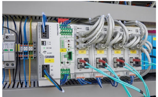
The 2200 series Managed Switches incorporate various redundancy mechanisms and security functions.
