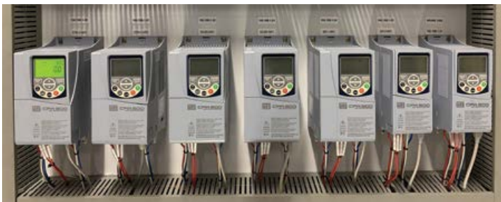
These WEG variable speed drives can prevent equipment from tripping out during loadshedding.
