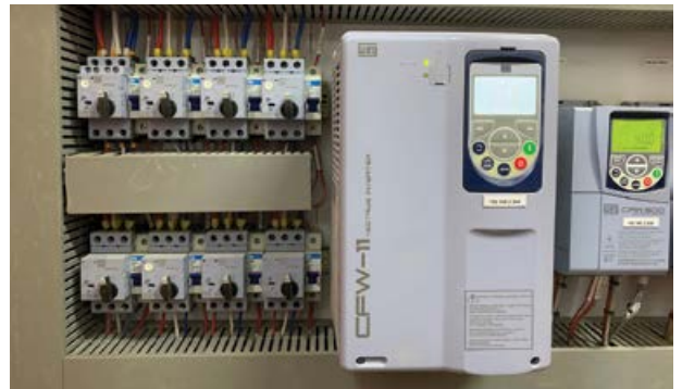
WEG variable speed drives with built-in PLC capability can be used to restart motor-driven processes smoothly.
