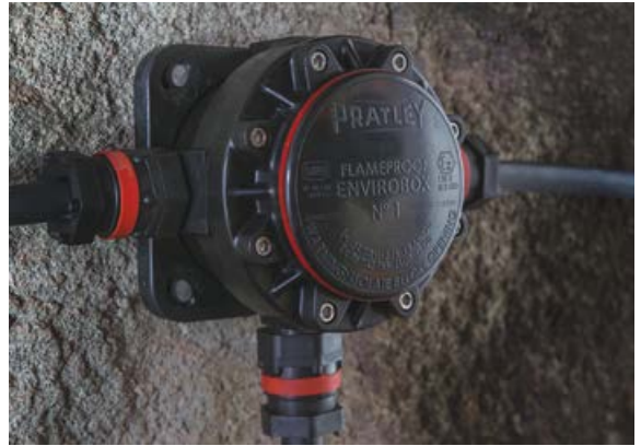
Pratley's new Flameproof Ex d Envirobox® junction box in an underground mining application.
