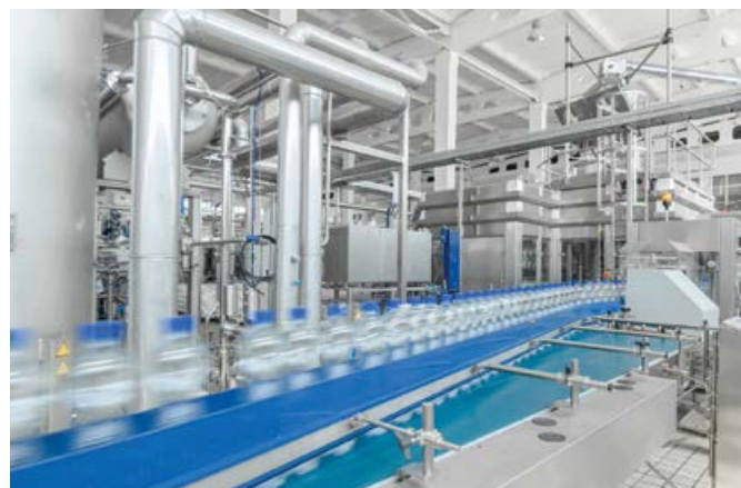
A DCS serves as the hub of a process operations and controls, monitoring key variables.
