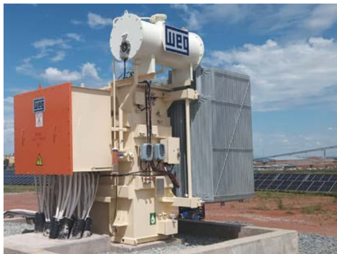
The LV termination side of WEG transformers is designed for maximum safety and reliability.
