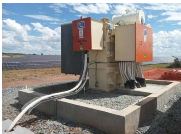
The MV and LV terminal boxes of the 5 MVA PV transformers.
