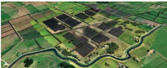
Lodestone Energy selected Emerson's automation and control technology for New Zealand's first large-scale solar PV plant.
