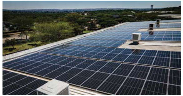
Solar panels installed on the roof of Yanfeng's plant in Rosslyn, Pretoria.
