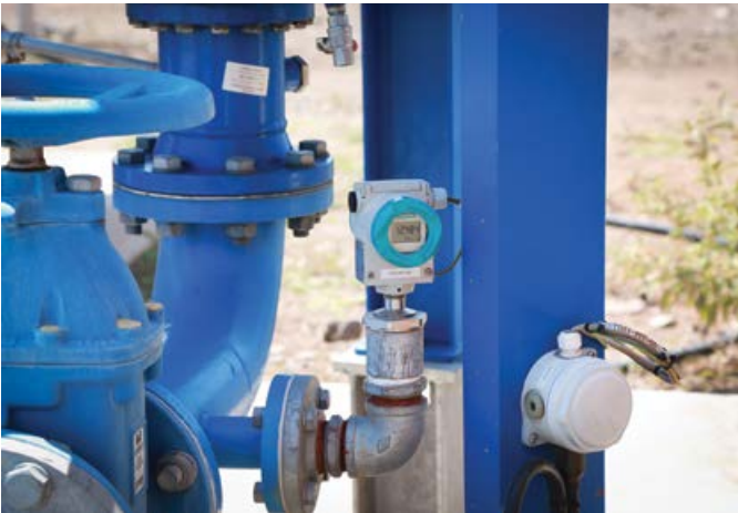
Monitoring water levels and water flow at Thune Dam.
