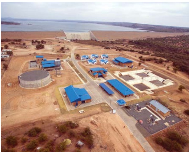
The water supply works at Thune Dam, Botswana, one of the infrastructure projects Siemens was involved in recently.
