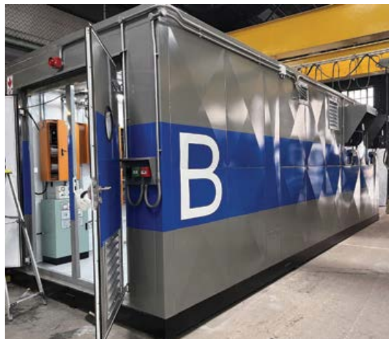
Modular substations reduce the need for on-site work, reduce project time and save money. This modular substation was custom engineered for a data centre application.
