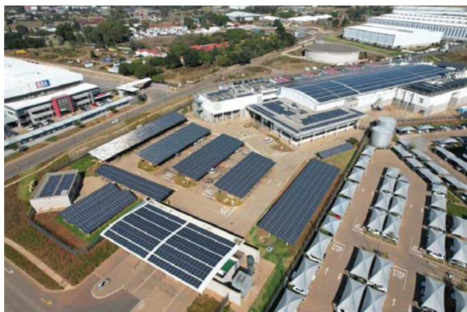
Teraco has already installed a solar PV energy system at its JB2 facility in Isando.
