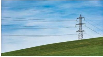
Power factor correction and voltage optimisation can enable savings on energy costs.
