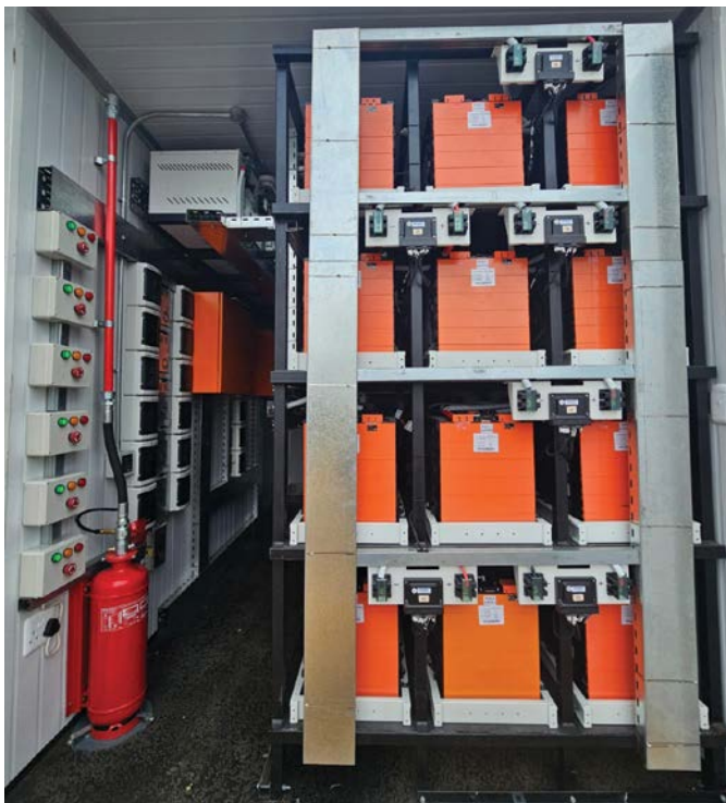
BESS installation at Inyati Lodge.
