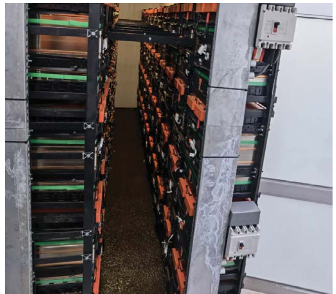
A containerised HV battery energy storage system.
