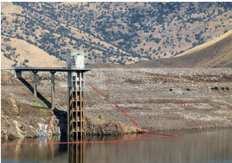
Communications systems for remote water reservoirs often need to traverse craggy or mountainous terrain to share monitoring data with the water management control station.
