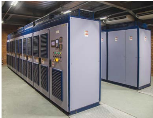
WEG medium voltage variable speed drives operating in a mine.
