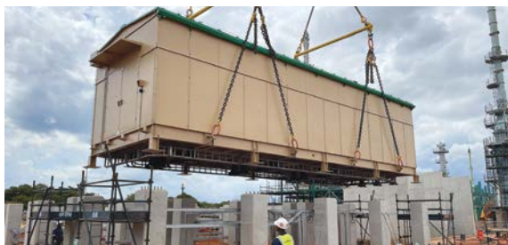
Rigging the first WEG E-house pod into position on the project site.
