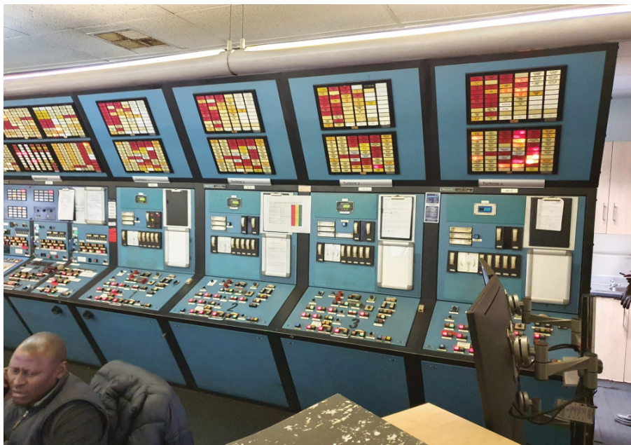
Maxiflex pole-mounted RTUs are interfaced to a central control room, to enable remote monitoring and resets when necessary.
