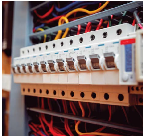
ELPDs monitor the flow of current in a circuit and trip when they detect even a slight imbalance.
