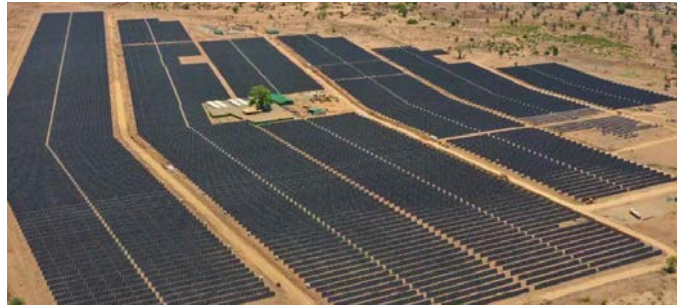
Africa's drive towards renewable energy is intensifying and there is a growing need for solutions that enable faster, smarter, and cost-effective utility-scale solar PV development.
