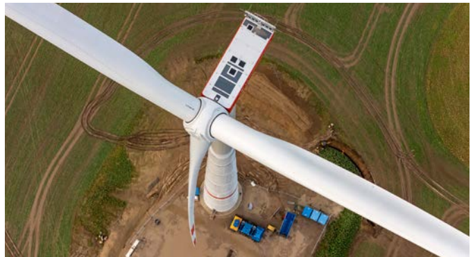
The N175/6.X wind turbine developed by the Nordex Group has a hub height up to 179 metres.
