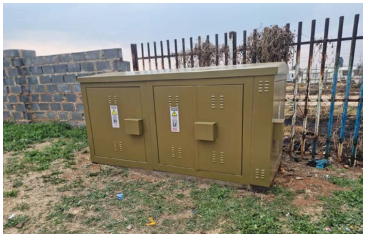
Before and after photos illustrate a previously damaged mini substation completely refurbished with renewed outer shells, repaired inner works and enhanced security features.
