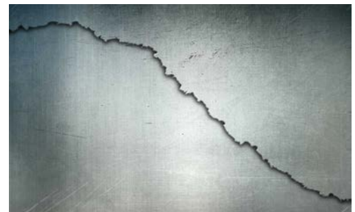
DEKRA Industrial's advanced testing services include inspection services to detect hydrogen-induced cracking in steel vessels.
