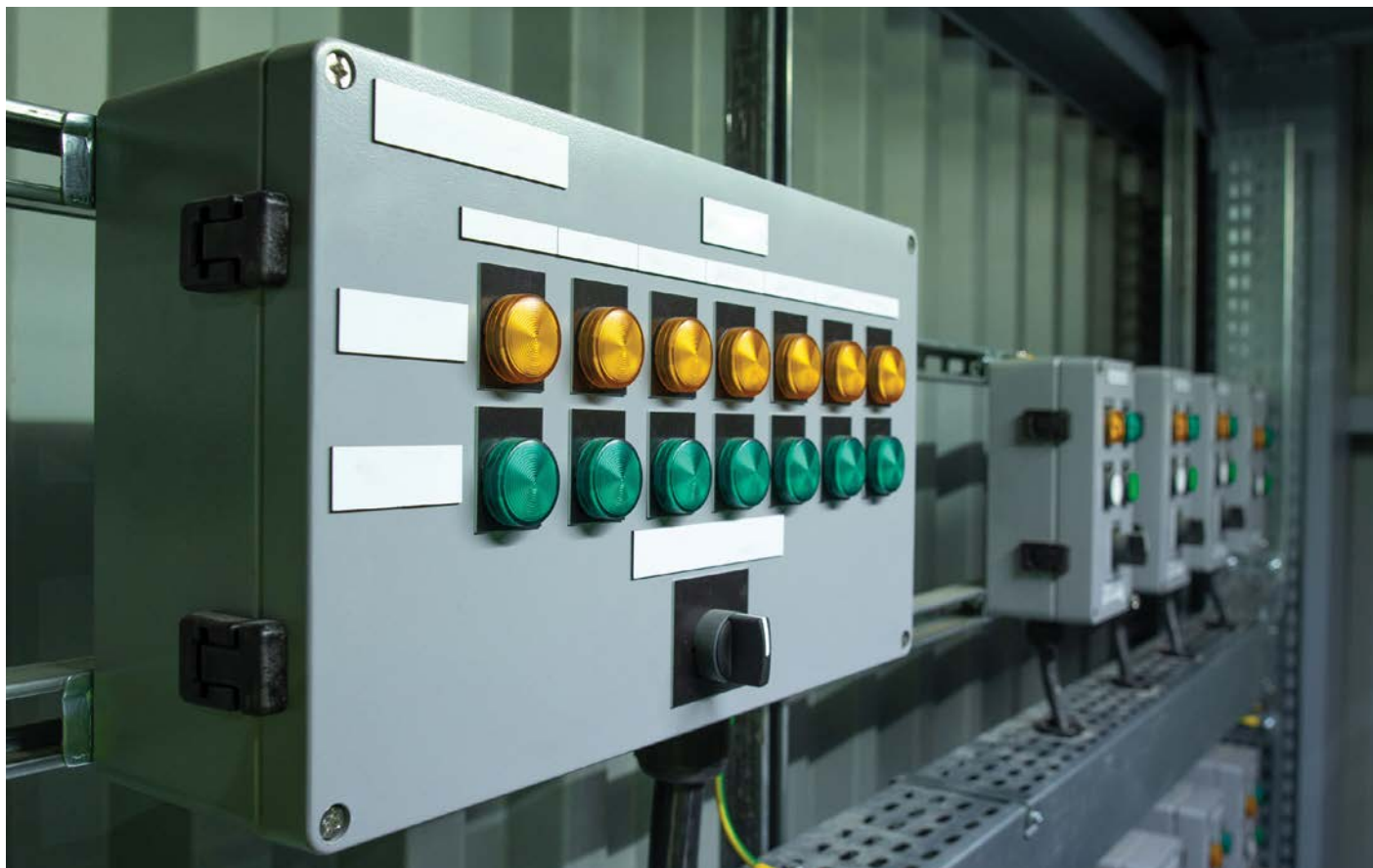
EC&I construction teams handle the last stretch of a project: installing the electrical systems that provide power across the site.
