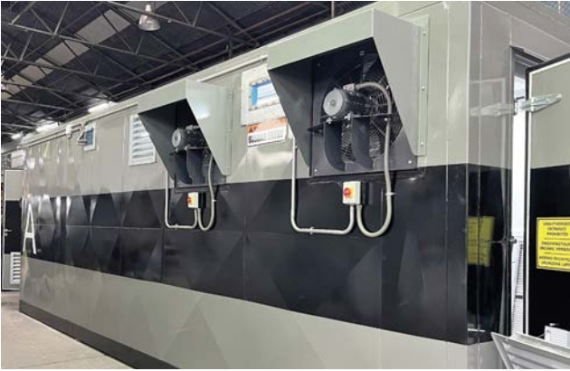
Cooling system designed by Trafo Power Solutions for a modular substation to maintain optimal temperature control and safe operation of electrical equipment.
