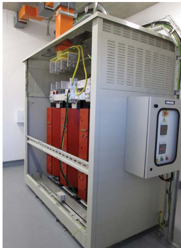
A dry-type transformer solution from Trafo Power Solutions with integrated control and protection,
