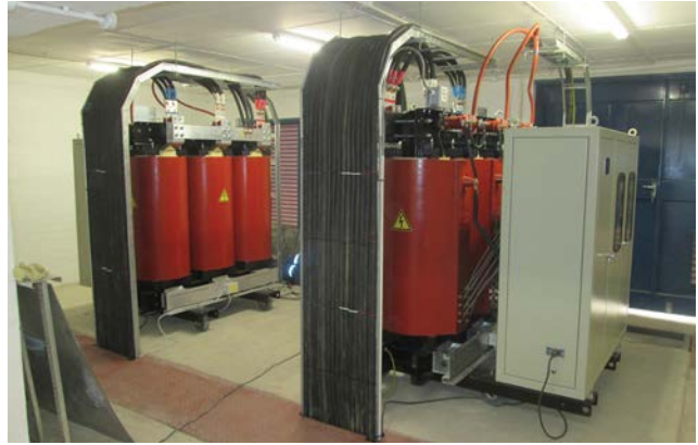
A dry-type transformer installation equipped with an On-Load Tap Changer to allow precise voltage regulation and continuous adjustment under load conditions.
