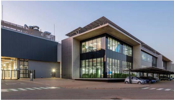
The total JB4 facility comprises 14 data halls with a floor area of 17 000 m 2 .
