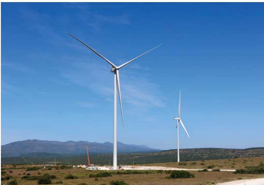
The Umoyilanga Dassiesridge wind farm, currently in construction, includes battery energy storage and a main transmission substation.
