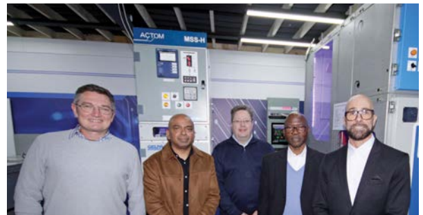
From left: Rhett Kelly, Design & Development Manager at MV Switchgear; Mervyn Naidoo, Group CEO; Johan Jordaan, Technology Development Specialist at MV Switchgear; Andries Mthethwa, Group Chairman; Donovan Stevens, MV Switchgear Divisional CEO.
