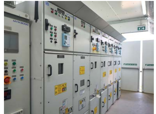
As modular, prefabricated units, each E-house is designed, assembled, equipped and fully tested to clients' and IEC benchmarks – enabling fast installation and commissioning on site.
