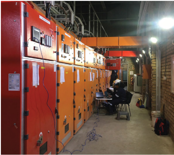
Testing and commissioning a UniGear Digital switchgear installation.
