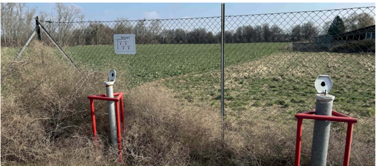
Measuring sites of the groundwater level on the extensive works premises and surrounding landfills.
