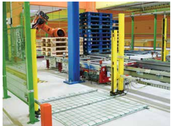
The safety of personnel is assured with Leuze sensors ensuring safe access.
