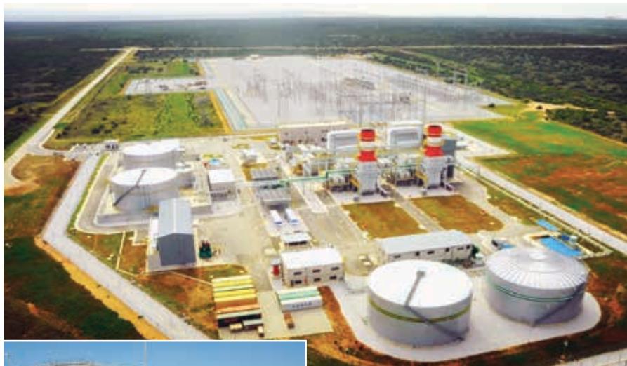
The Dedisa Power Peaking Plant, a 342 MW open cycle gas turbine power peaking plant located in the Coega SEZ, has attracted R3.5-billion in foreign direct investment.
