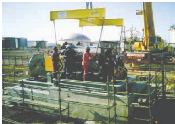
The KSB Pumps and Valves team lowers the diesel engine into position on installed baseplate for alignment with gearbox and pump.
