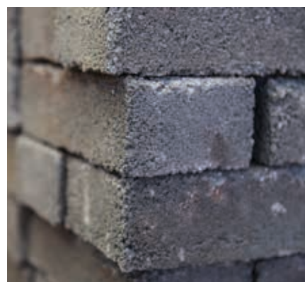
The brick looks and feels like a cement brick, however no water or cement is used in the production of the bricks.
