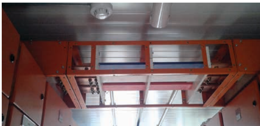
The busbar trunking support bridge mounted to the roof of the container.
