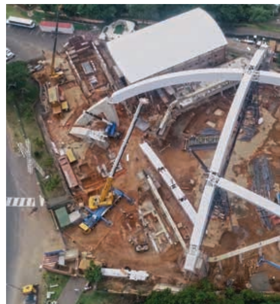
The innovative design of the Durban Christian Centre lay in the geometry of the large roof arches, inclined in different planes, which provide support for the roof as well overcoming tight site access issues. Inset: A view of the complex structural detail of the steelwork for the Durban Christian Centre’s roof.
