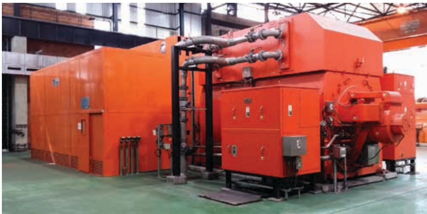
A turbo generator installed in a paper mill in South Africa.
