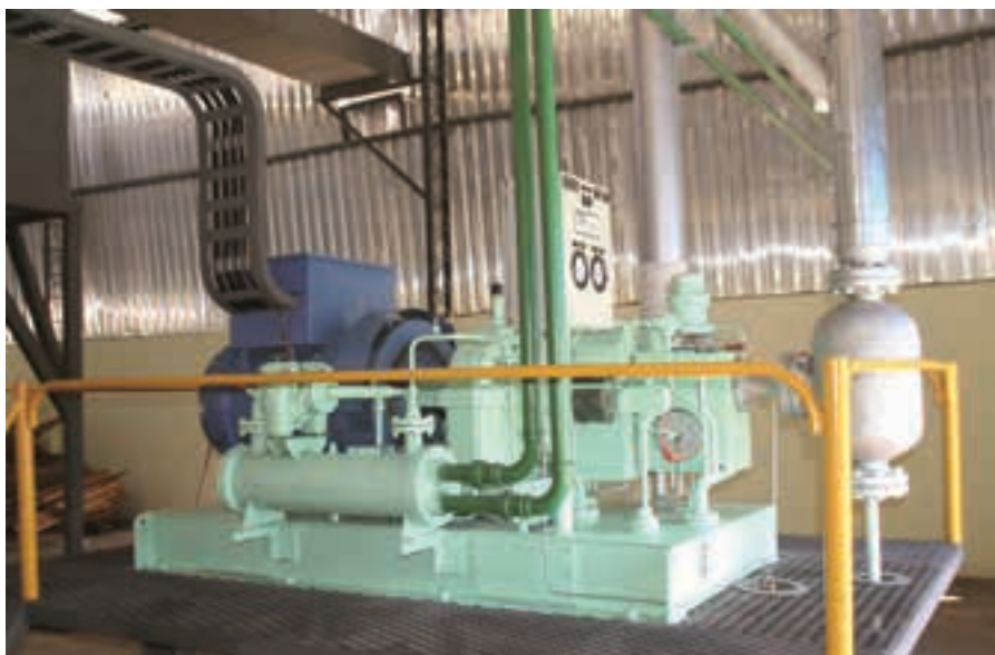
A backpressure steam turbo generator running with saturated steam, producing 100 kWh electricity to the plant.
