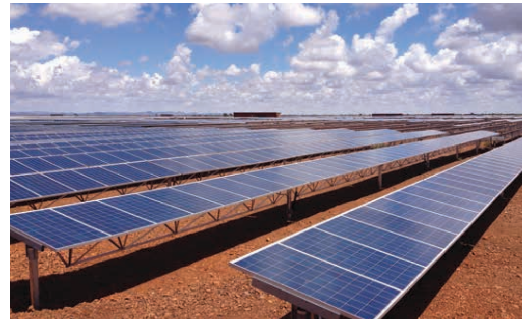
The Kathu Solar Energy Facility in the Northern Cape, which has an installed capacity of 100 MW and a 75 MW PV system mounted on a tracking system to follow the sun throughout the day. Kathu owners Reisa and Building Energy appointed Aurecon as owner's engineer to ensure technical compliance on all civil, electrical and construction issues, and to assist with the resolution of technical queries and disputes.
