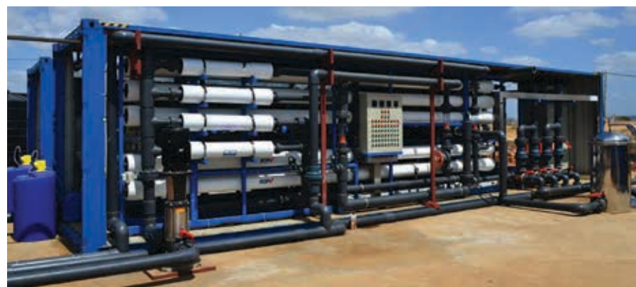
Aquamarine has a long history of producing desalination units for farming, industrial and commercial use, mostly small to medium sized membrane-based plants that could be quickly deployed.
