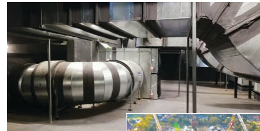
Above: The total cooling load is 3.2 MW, serving 17 AHUs catering for different thermal zones.
