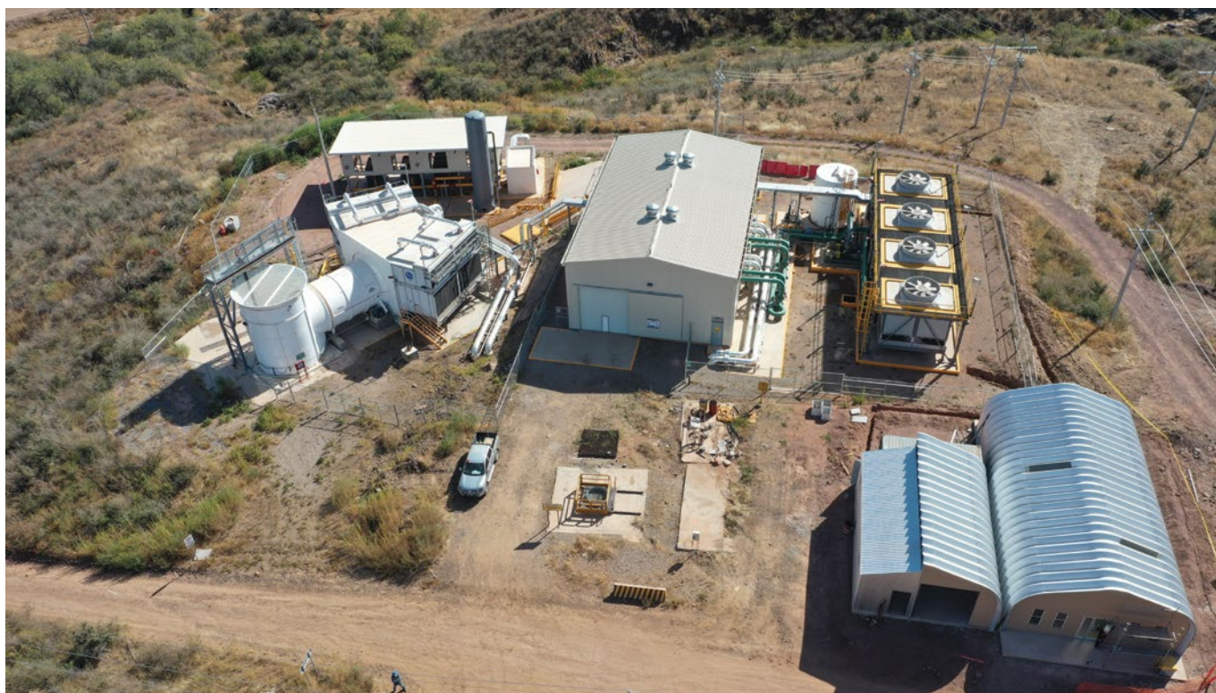
The main fan stations are dual axial fan systems with a total air flow of 240 m 3 /s at a total pressure of 1.8 kPa.
