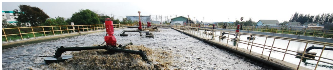
SEW-EURODRIVE is supplying 20 of its MC Series parallel shaft industrial gear units (inset) for the aeration tanks of an upgraded wastewater treatment plant in the Western Cape.
