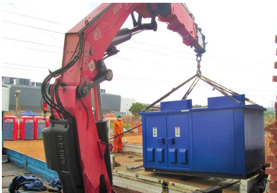
A 500 kVA dry-type mini substation being lifted into position at a commercial building site.
