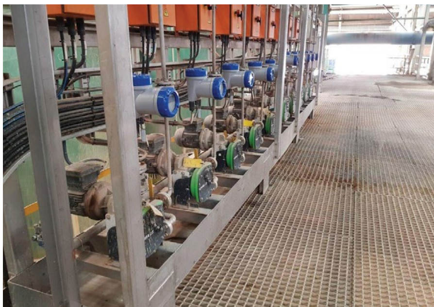
On the copper mines in DRC, racks of Dura 25 hose pumps are being used to dose reagents at massive flotation plants. These pumps can also far more efficiently manage dosing applications at wastewater treatment plants.
