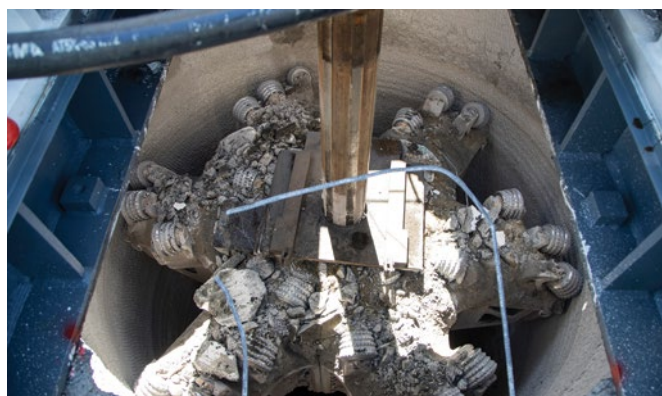
At 1 380 m deep, Shaft 3 at Zondereinde in the Limpopo Province of South Africa has set a new world record for the longest raise bore shaft ever built.
