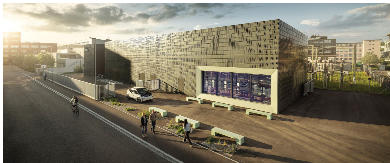
The step towards ABB's Mission to Zero is to deploy digital solutions for smart green buildings and energy management, such as monitoring, control and optimisation.
