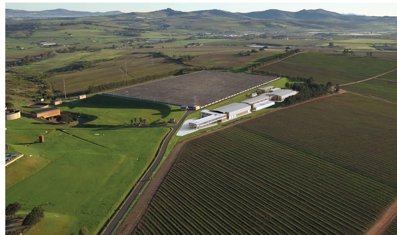
An aerial view of the Zutari-designed Faure New Water Scheme, a new flagship direct potable water reuse project.
