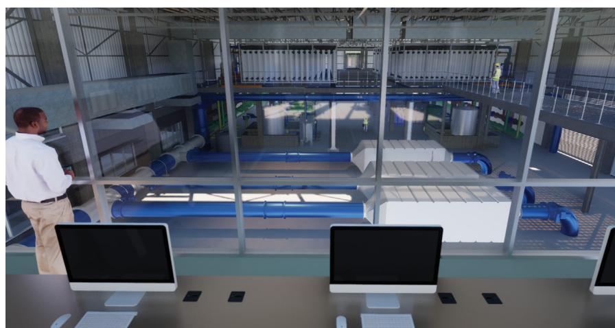
The control room at the end of the treatment process overlooks the UV-based advanced oxidation process (AOP) that breaks down any remaining organic chains into CO 2 and water.
