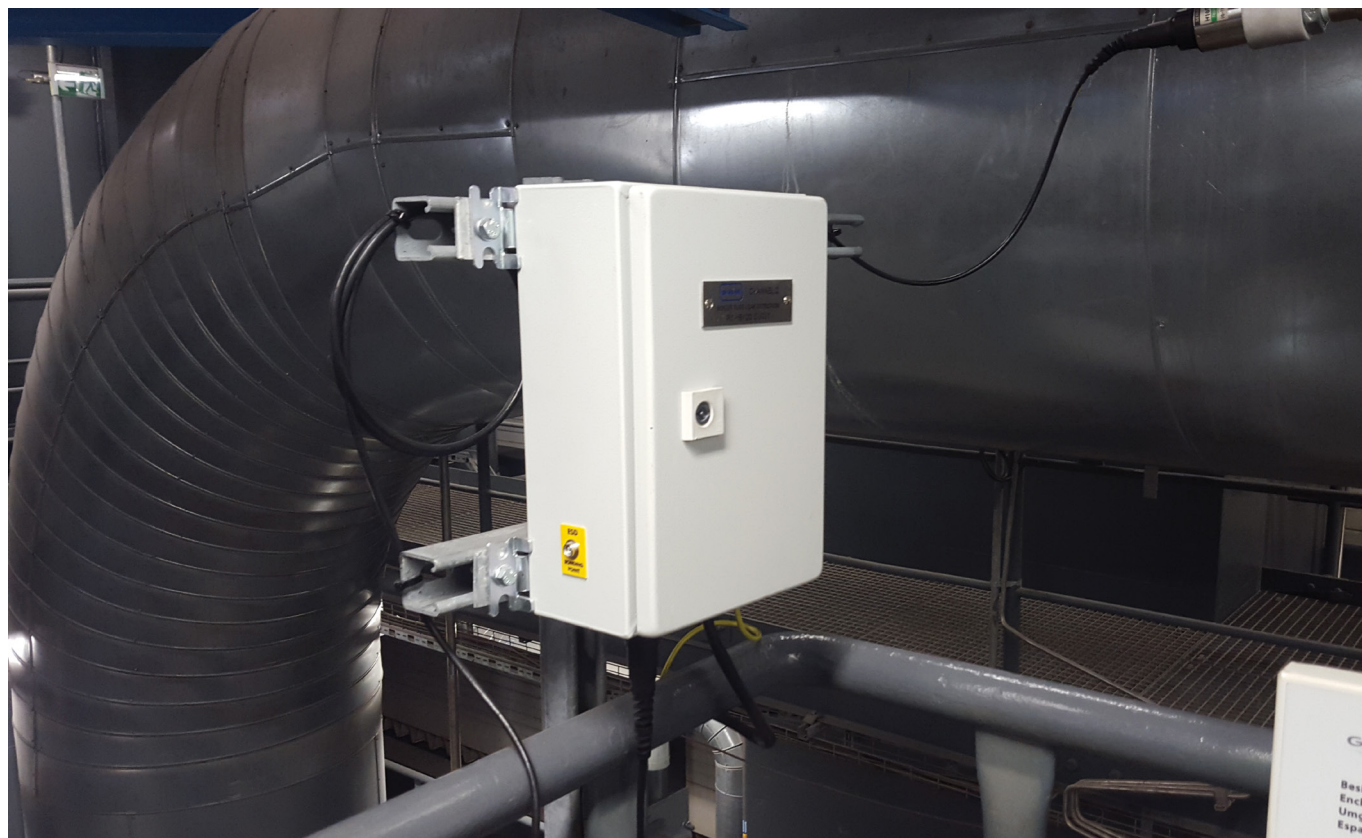
Procon’s early warning boiler tube leak detection system is based on the use of acoustic and structure-borne sensors to pick up operational changes within working boilers.
