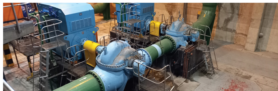
A bulk water supply company pumping station that uses pumps in parallel to deliver water to multiple destinations. Each destination change results in changes to the system pressure profile and the operating points of all the pumps.
