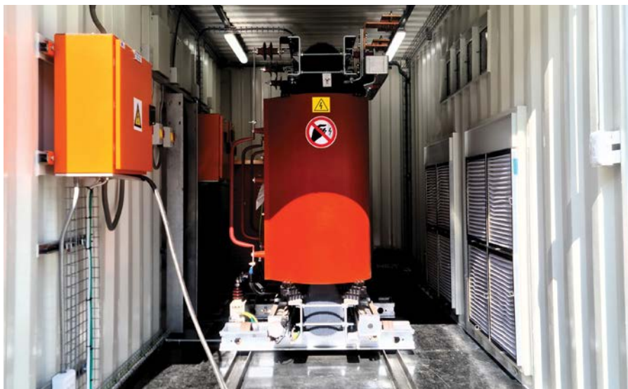
A 3 000 kVA dry-type transformer supplied by Trafo Power Solutions is housed in a modular substation, providing a robust and efficient power solution tailored for demanding site conditions.
