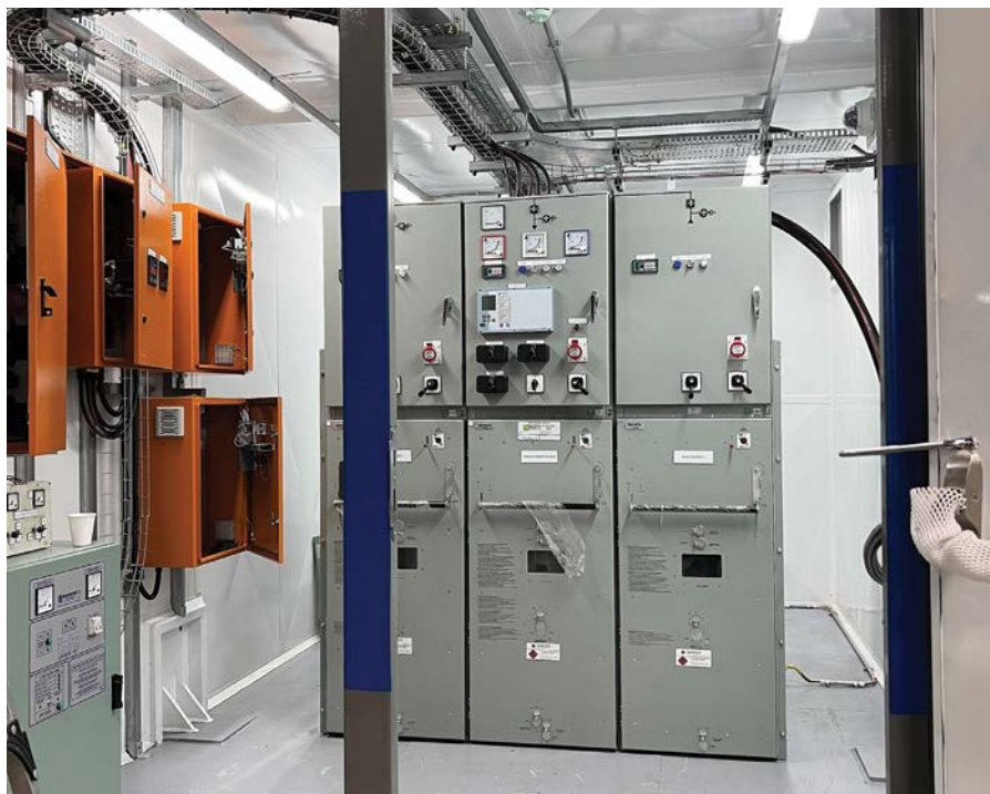
A Trafo Power Solutions dry-type transformer paired with 800 A primary switchgear within a modular substation, a factory-assembled, robust power package ready to deploy on site.
