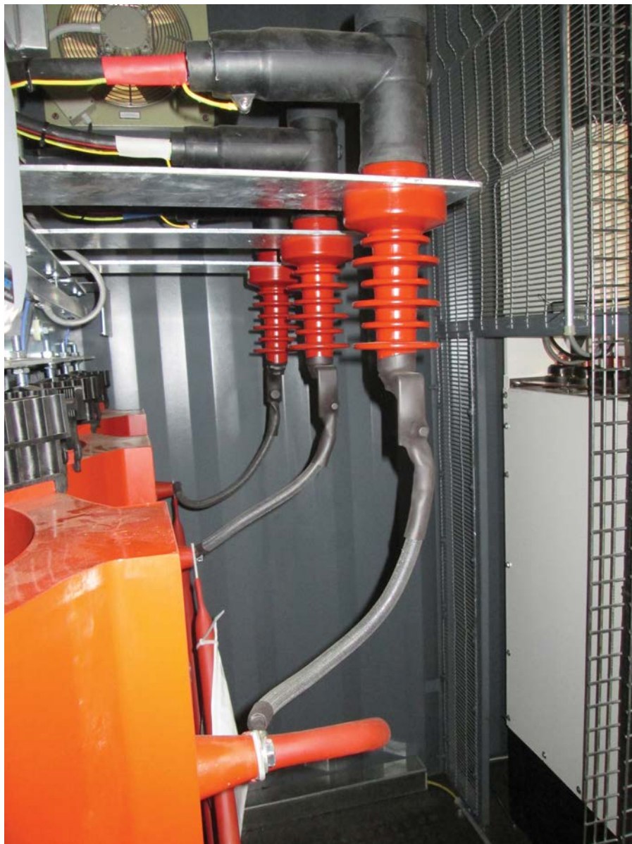
A dry-type transformer supplied by Trafo Power Solutions is installed within a modular substation, delivering safe and reliable power distribution for this application.
