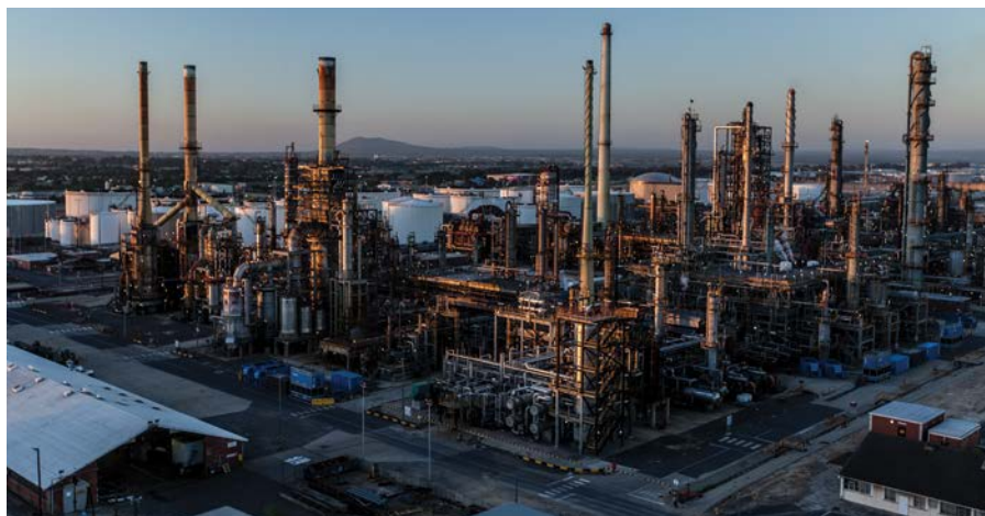
The Astron Refinery in Cape Town is one of South Africa’s last remaining major oil refineries.
