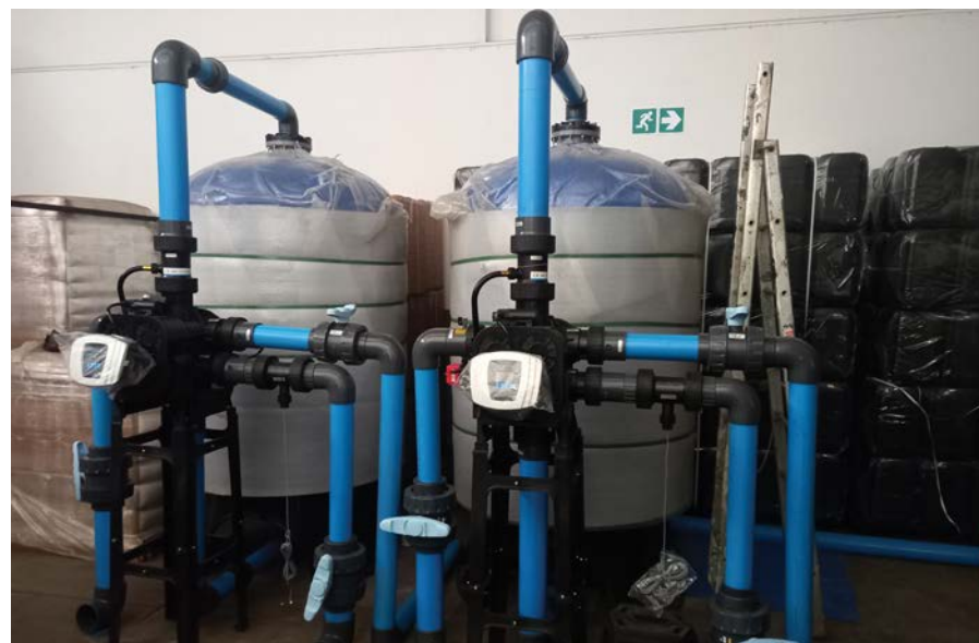
Sizing a boiler water treatment and filtration plant based on accurate data yields better results than relying on guesswork, saving unnecessary expenses due to downtime and expensive repairs.
