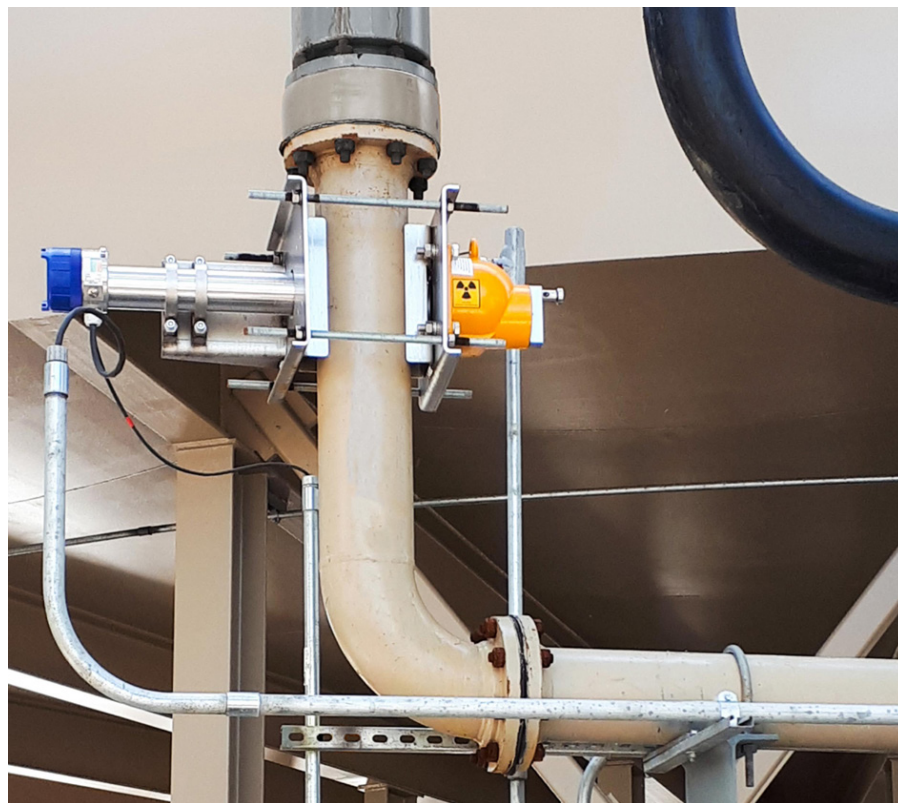
A SmartSeries Berthold LB414 radiometric detector continuously monitors the underflow density of a thickener.
