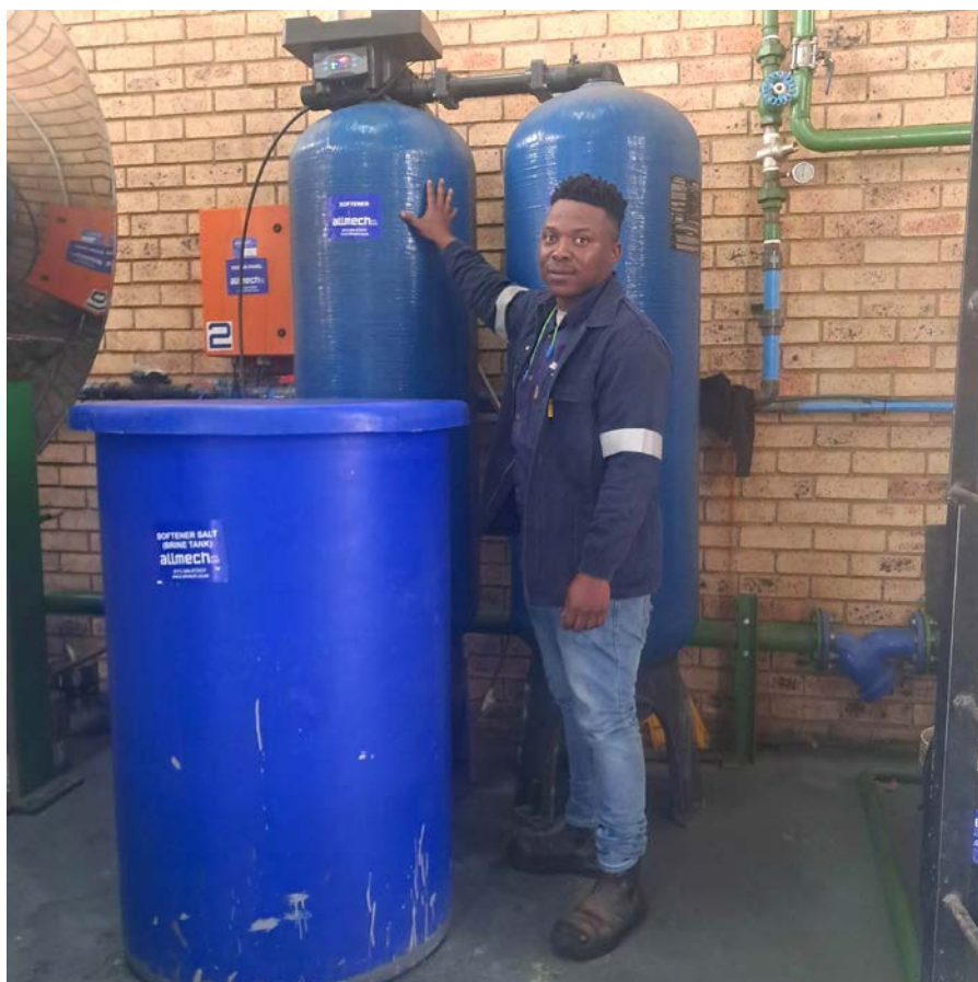
"We chose the F135 because it's a true duplex system that uses a single valve to control both of the softening supply vessels," explains Lucas Makgopa, one of Allmech's water treatment technicians.
