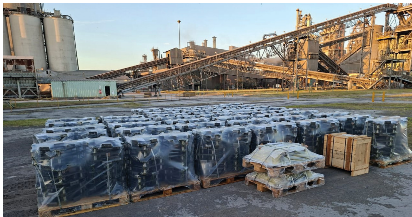
Bi recently installed a high-performance Kobo dual/double-chain pan conveyor in the cement industry, a first-of-its-kind installation in South Africa. Kobo heavy-duty chains can enhance reliability, efficiency and longevity.
