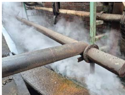
Left: Steam line offtake design is critical to ensure no condensate pickup. Middle: Wasted condensate from the steam trap is discharging to the ground. Right: Thermal images of steam traps are used to assess their functionality.
