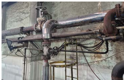
Left: Steam line offtake design is critical to ensure no condensate pickup. Middle: Wasted condensate from the steam trap is discharging to the ground. Right: Thermal images of steam traps are used to assess their functionality.
