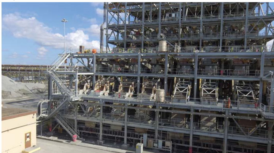
Eccentric technology virtually eliminates vibration in the extended structure, which protects the integrity of the screening machines.
