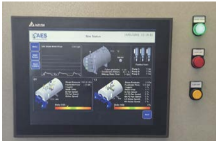
Remote monitoring system (RMS) platforms allow operations management to monitor performance, investigate anomalies and conduct detailed root cause analyses
