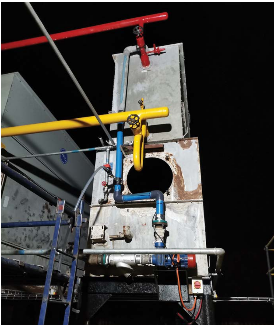
Bleed, or blowdown, is the process of removing a portion of high-TDS (total dissolved solids) water from the system and replacing it with fresh make-up water.
