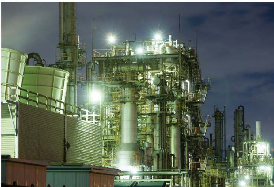
Babcock recently completed a fast-tracked industrial boiler upgrade project at a major South African refinery.
