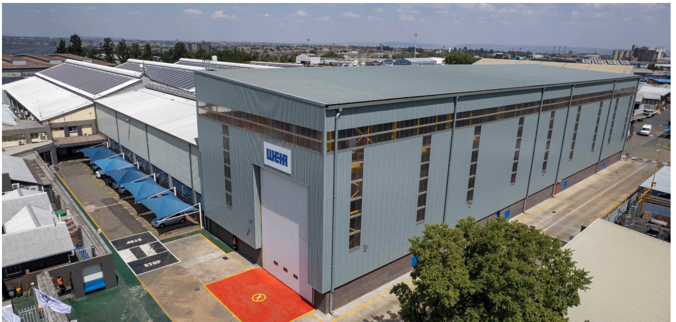
The recent expansion at Weir Alrode, which included the addition of a heavy bay screen manufacturing facility, has added a further 1,600 m 2 of dedicated production space under roof.
