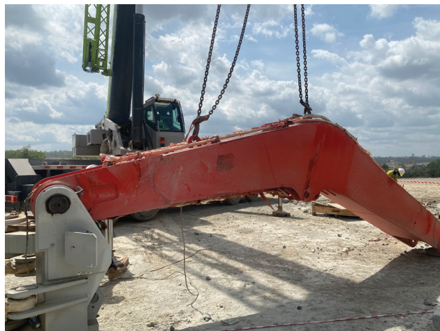
Left: Installation of the refurbished Sandvik BR3288i hydraulic breaker and BB8094R breaker boom has been completed, and the unit is now ready for testing in the primary crushing circuit. Right: Coupling of the main boom to the pedestal is underway as part of the Sandvik rock breaker installation.
