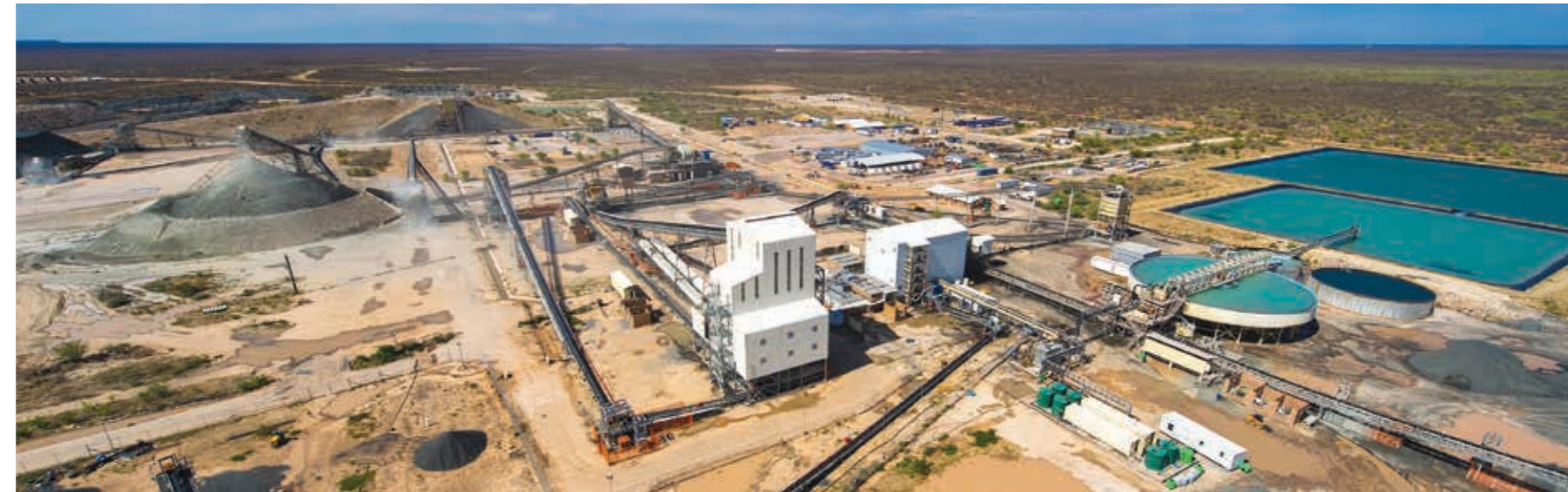
A view of Lucara's Karowe mine in the Orapa Kimberlite Field of Botswana. The tall building in the centre of the photo houses the XRT sorters (photo: Lucara).
