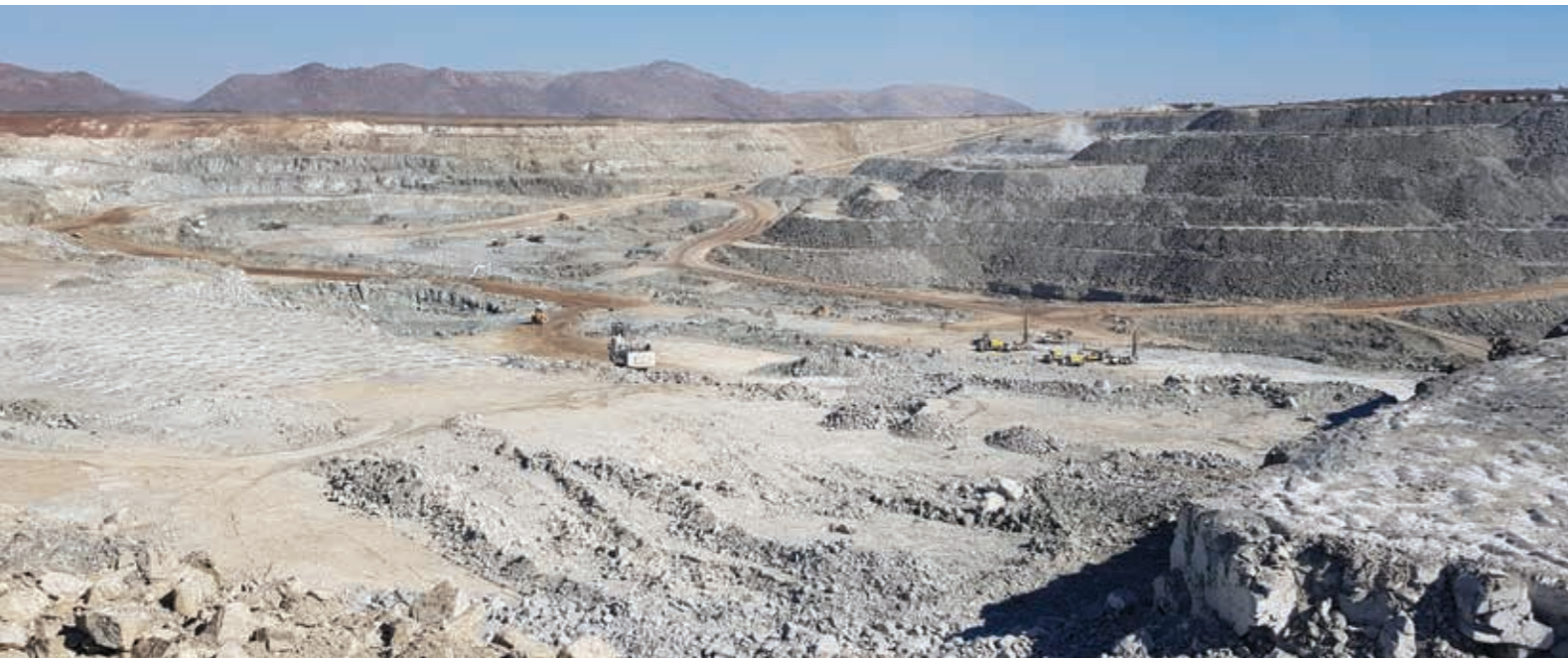
Preparations for the first CE4 Commander™ trial blast.
