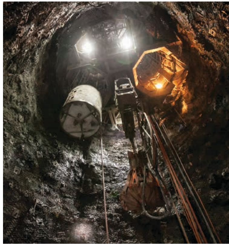
Sinking platform in operation at Shaft 1 (photo: Ivanhoe).
